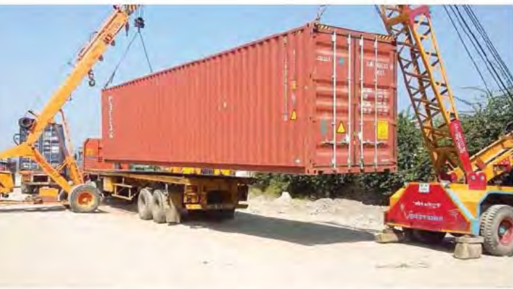
Logistics Plus India spent significant time planning and coordinating to ensure all bridge equipment and parts arrived at the job site on time and intact.
